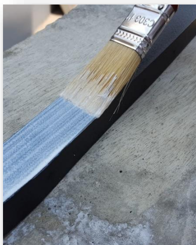
Apply Waterstop Delay Swell Coating on all exposed sides of waterstop
