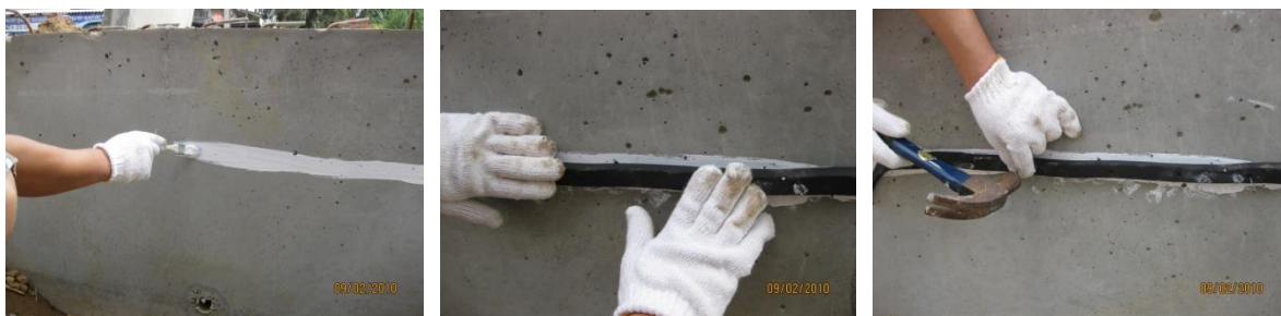
Fixing bentonite swelling waterstop on concrete surface
