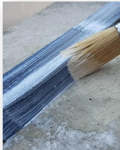
Apply Waterstop Delay Swell Coating on all exposed sides of waterstop
